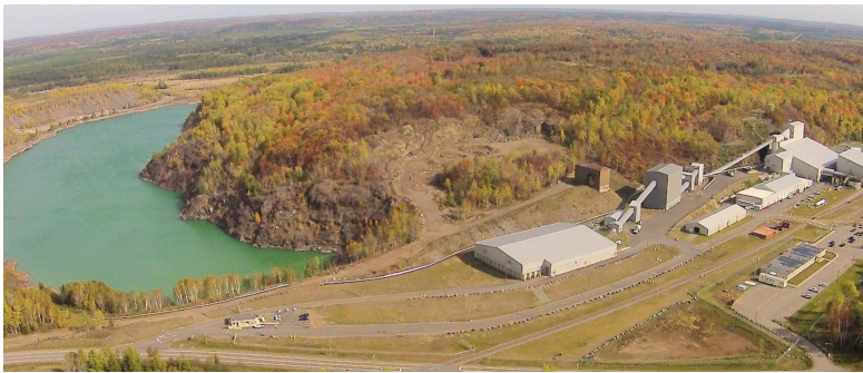
Lundin Mining's Humboldt Processing Mill and Tailings Disposal Facility serving Eagle Mine
